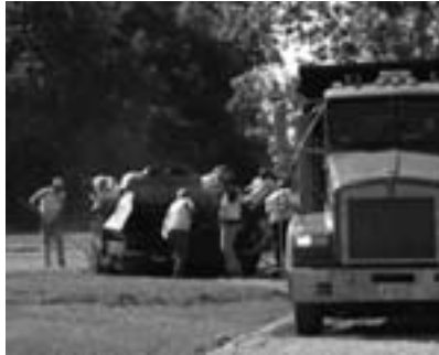
Building the new bike path.
